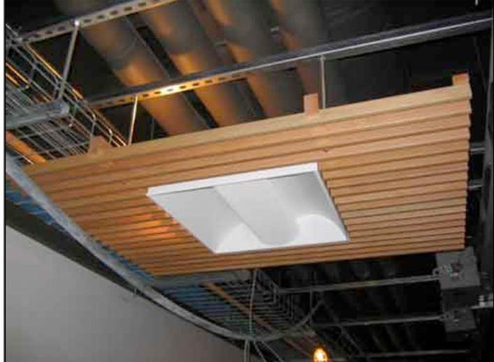
Simon Fraser University saved \$30,000 (CAD) by using cable trays for controls wiring in its new Technology and Science Complex 2. (Photo courtesy of Chernoff Thompson Architects.)
